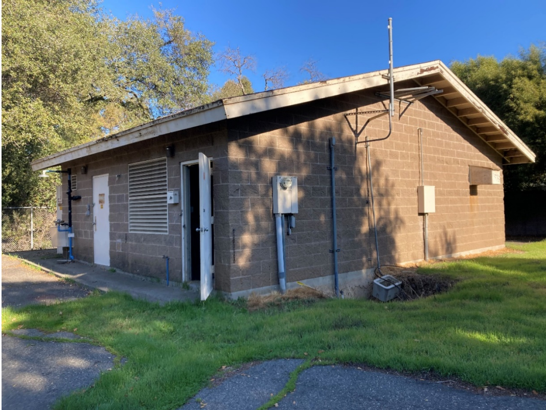
Chlorination facility, view from main entrance, main door open
