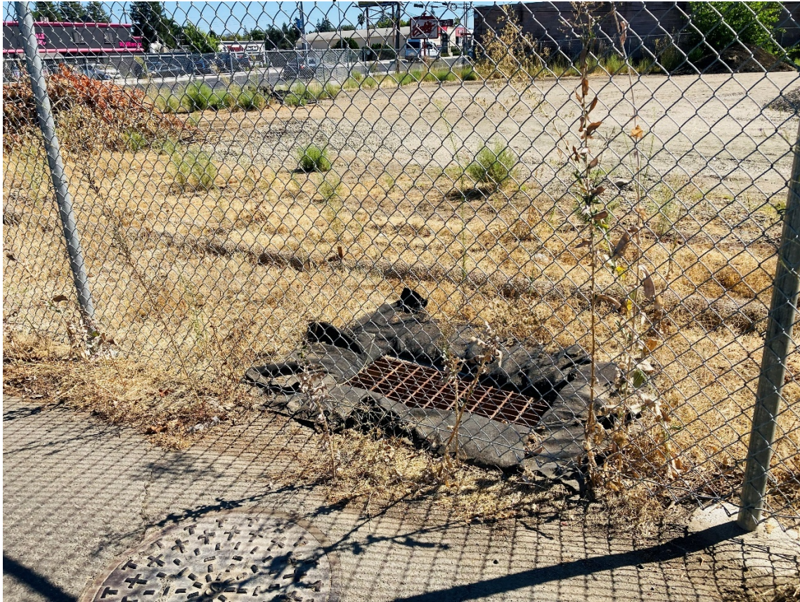
View from Angelina Ave Drain improvements installed
